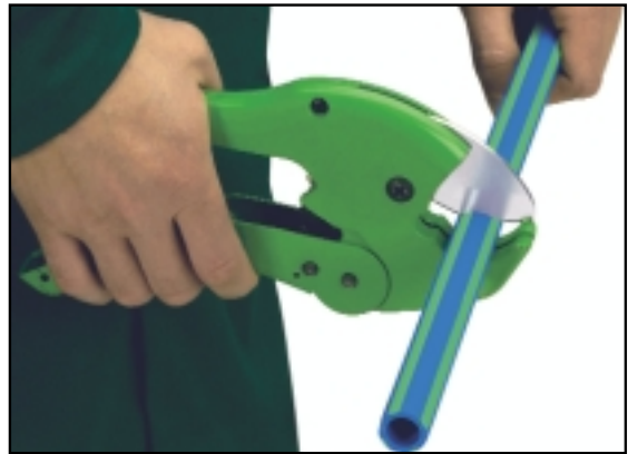
Cutting the pipe
