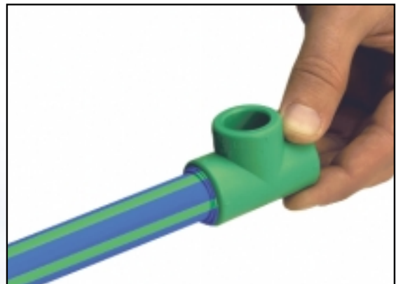
Fusioning, fixing and aligning of fittings
