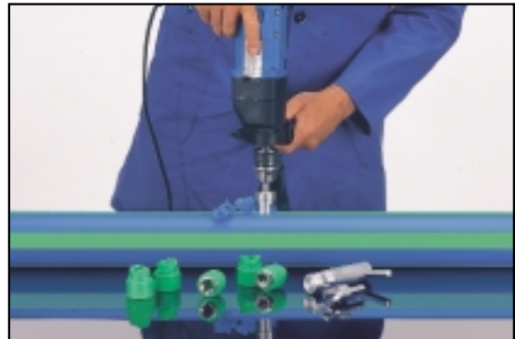
Drilling through the pipe wall
