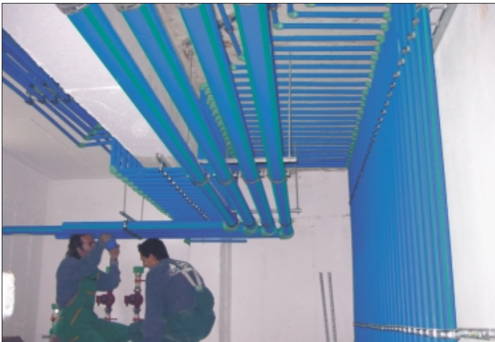
Installation of climatherm -pipe system
